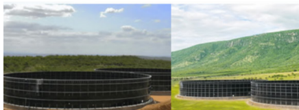
North America GFS-Landfill Leachate Tanks
